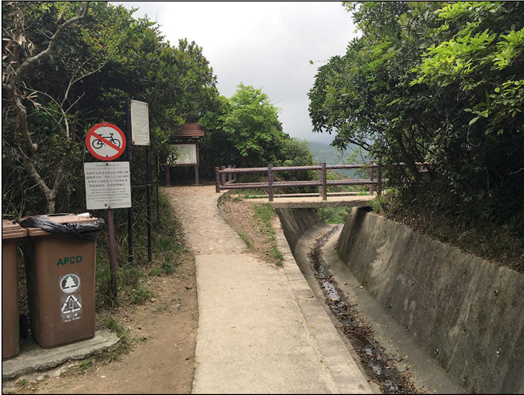
Figure 3. The Tsz Kong Bridge
